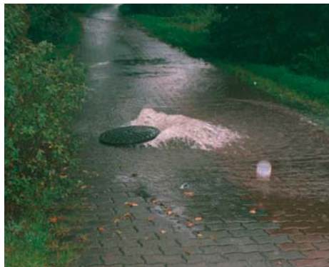
Overflow: water emerges from manhole
